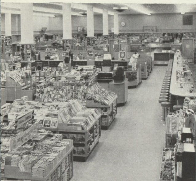
Mass display on self-serve counters encourage customers to buy. Interiors designed for easy and speedy shopping—help build volume at 801 16th St., Denver, Colo.
